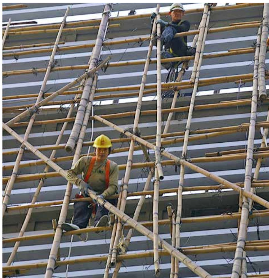
Bamboo scaffolding in use in Hong Kong: combining old and new materials
