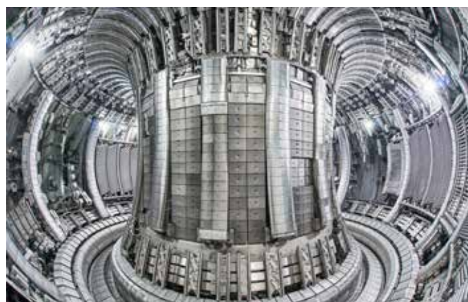
An internal view of JET with a complete metallic ‘ITER-like’ wall of beryllium and tungsten
