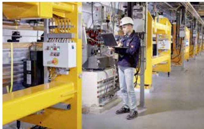
An engineer runs tests at the first fully installed undulator system in the European XFEL
