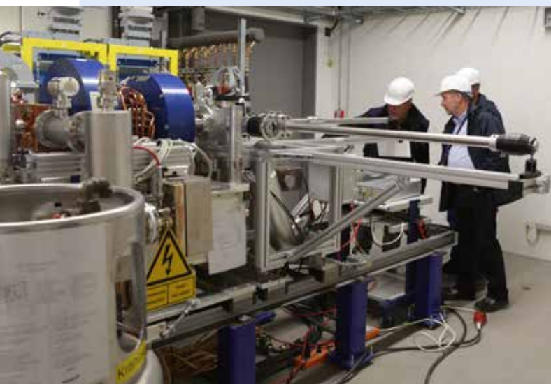
Workers prepare the European XFEL electron gun for installation.
