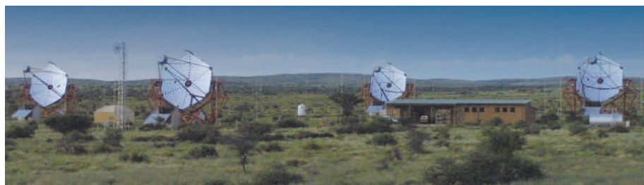
Figure 1 | Eyes to the light. The four HESS telescopes in the veldt of central Namibia.
