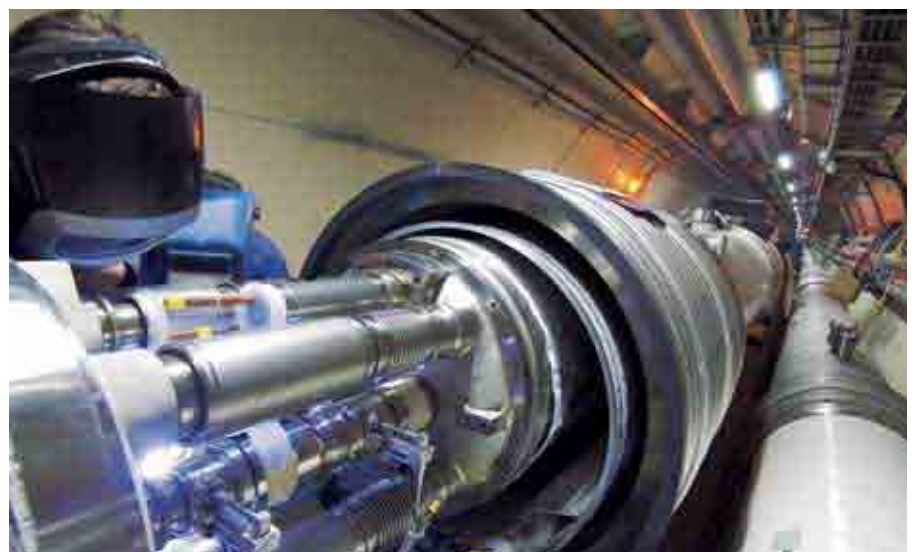
A welder making the very first interconnection between two cryomagnets for the LHC. The 1700 interconnections between superconducting magnets for the whole collider required 123 000 separate welding and assembly operations
